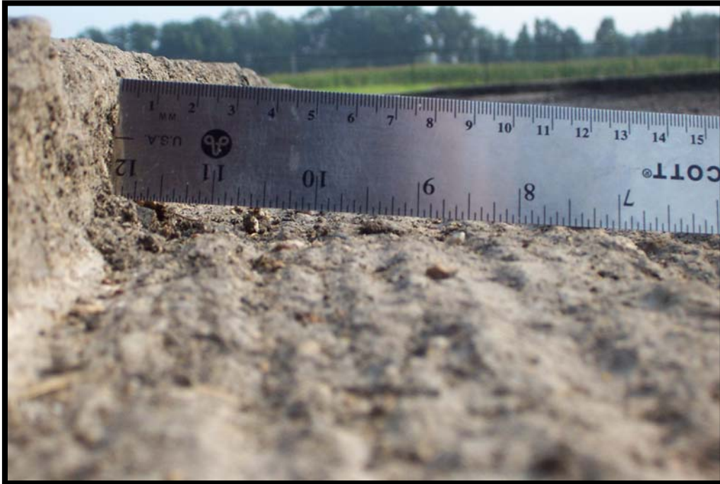
Figure 4.6. Milling pattern and texture depth using a milling head on a bobcat.
