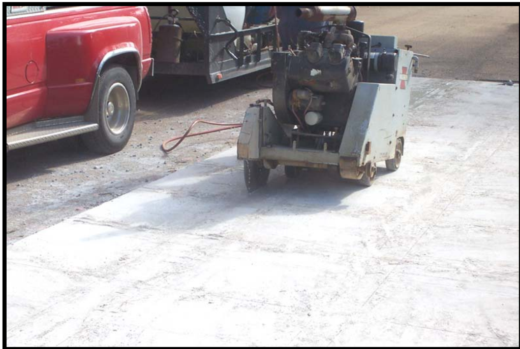
Figure 4.13. A Soff-cut® saw was used to cut joints at the test site.
