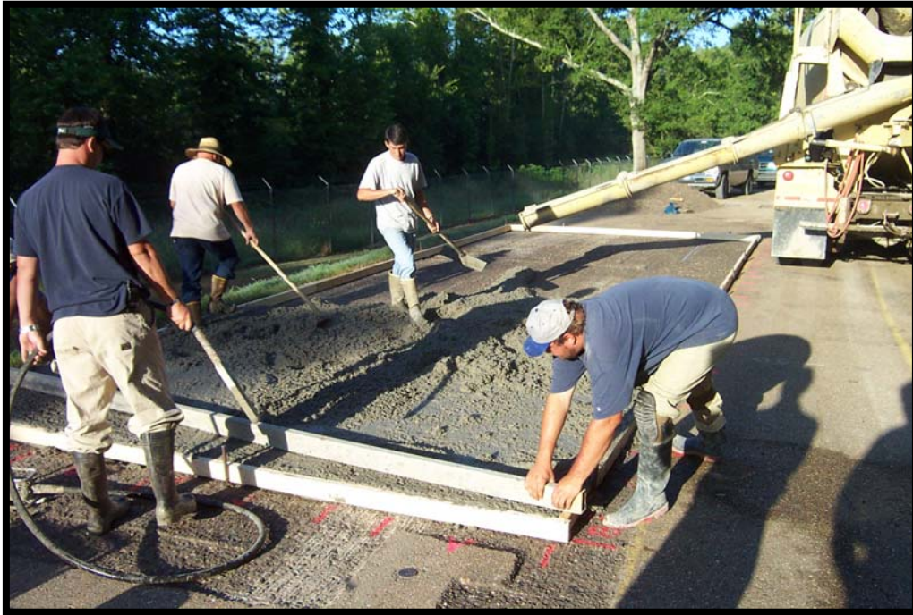
Figure 4.11. Concrete was manually placed and finished at the test site.
