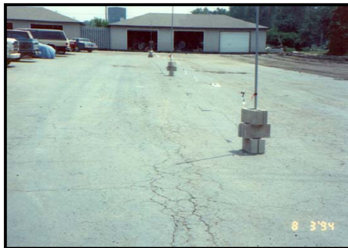
Figure 2.35. AC pavements at Holiday Inn parking lot exhibited alligator cracking.
