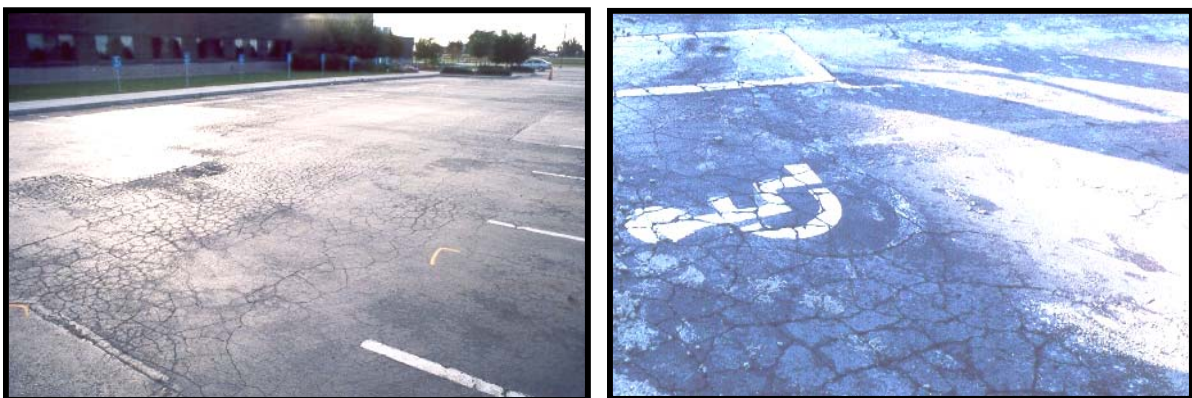
Figure 2.40. Life Bridge Christian Church parking lot was severely cracked.
