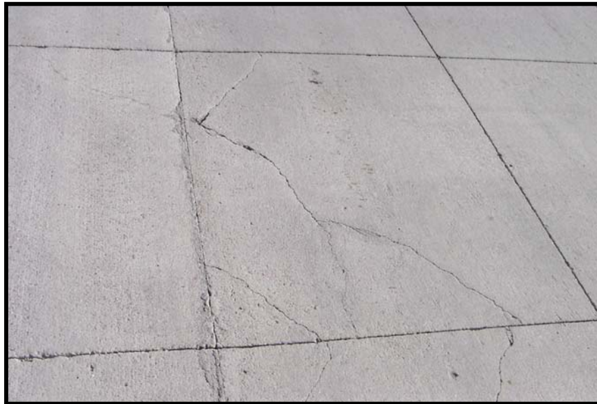
Figure 2.44. Thinner slabs led to premature failure.
