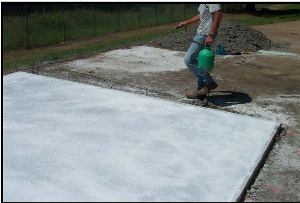
Figure 4.12. Curing compound was applied at twice the normal rate.
