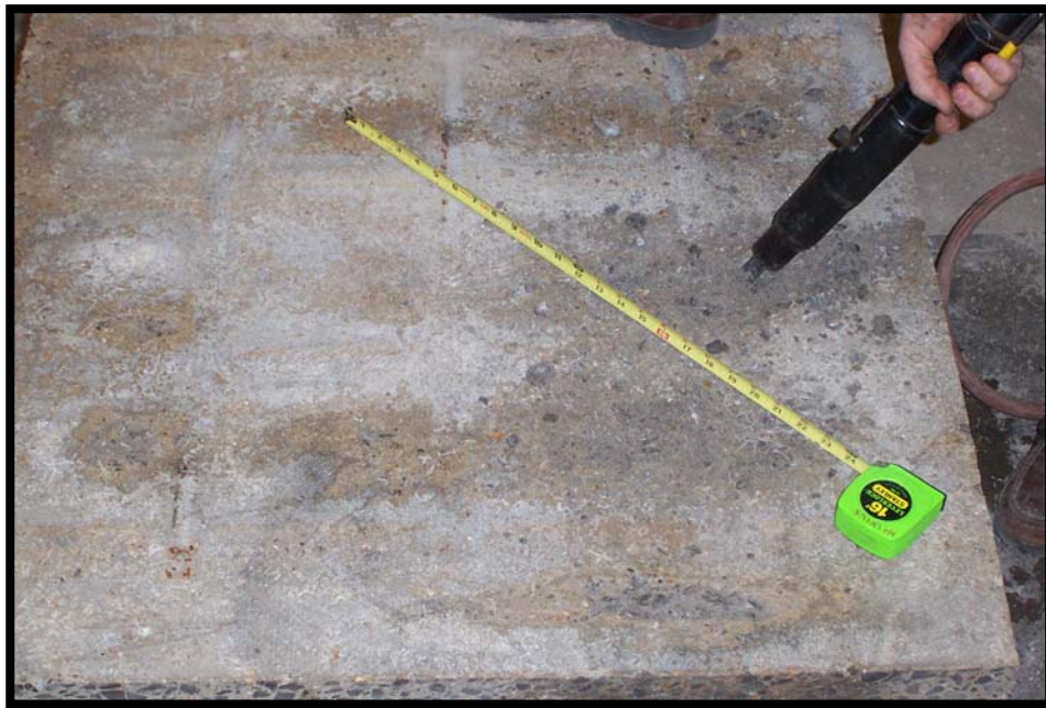
Figure 6.58. Severely deteriorated PCC surface was easily scrapped using a jackhammer.
