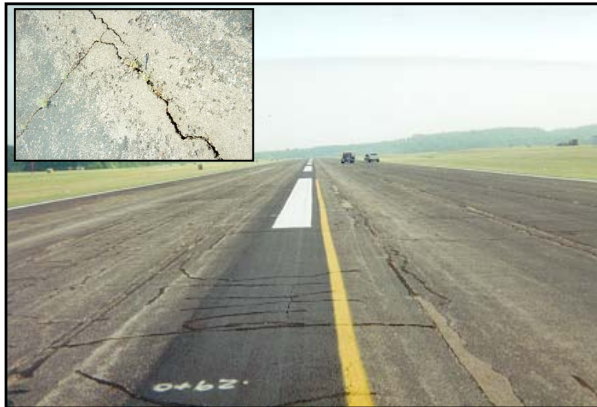
Figure 2.2. Block cracking observed on both sides of the runway centerline at SNH.
