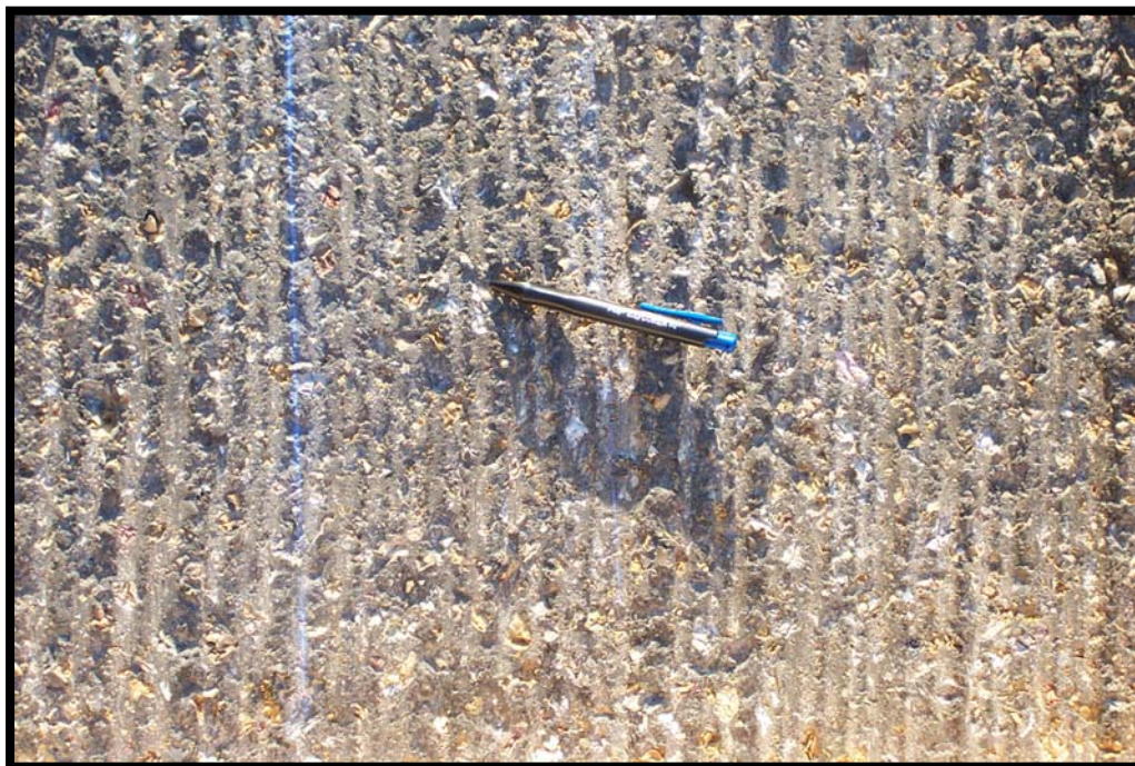
Figure 4.9. Milling at the test section resembled milling at a typical UTW project.
