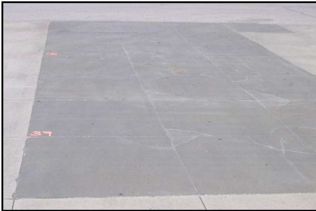
Figure 2.14. All slabs at the first left turn have corner cracks along interior joints.
