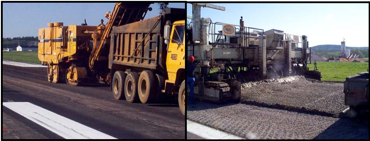
Figure 2.5. UTW placement at SNH followed milling of existing AC pavement.
