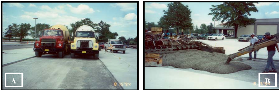
Figure 2.36. Slip form paver was used at the Holiday Inn parking lot.
