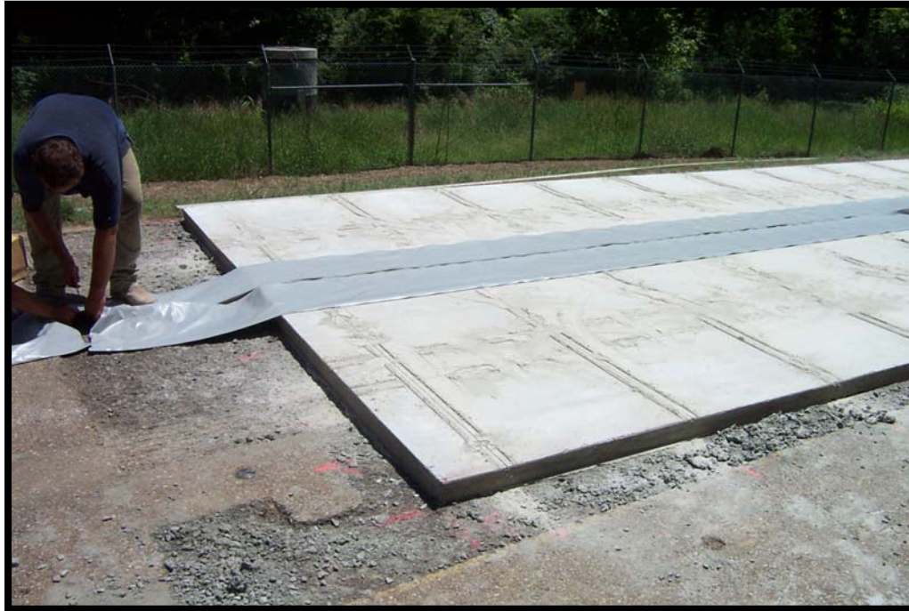
Figure 4.14. The PCC was covered with a plastic sheet after initial joint cutting.
