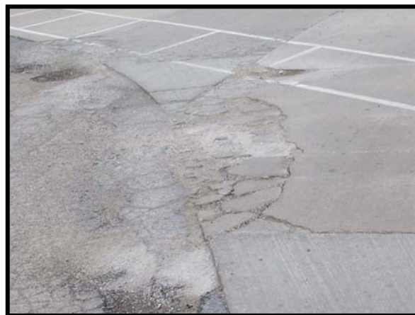
Figure 2.30. PCC Slabs on transition from AC to PCC were severely distressed.
