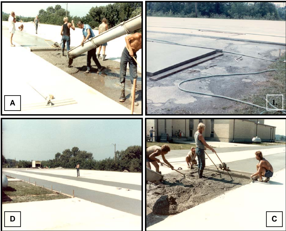
Figure 2.28. PCC was placed manually at Williamstown Jr. & Sr. High School.
