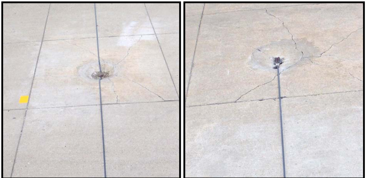
Figure 2.16. All slabs containing aircraft tie downs were shattered.
