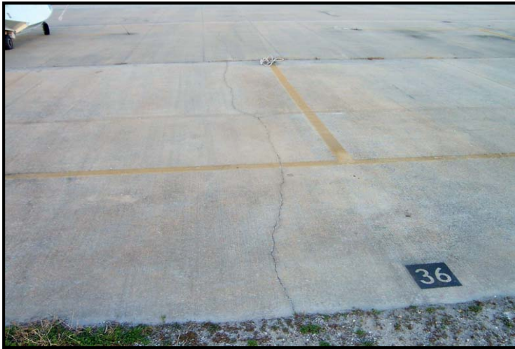
Figure 2.22. Large 26-ft by 13-ft (8-m by 4-m) slabs cracked into two pieces.
