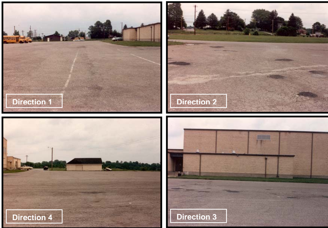
Figure 2.27. AC pavement at the Williamstown School was severely distressed.
