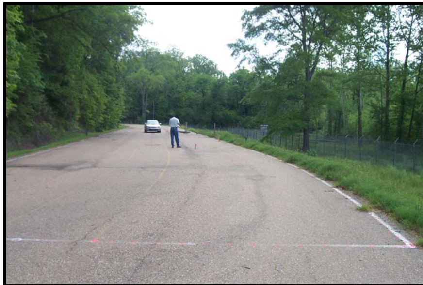
Figure 4.2. Approximately 125 ft (38 m) are available for test road construction.
