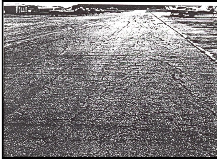
Figure 2.19. Alligator cracking of AC surface at New Smyrna Beach Airport.
