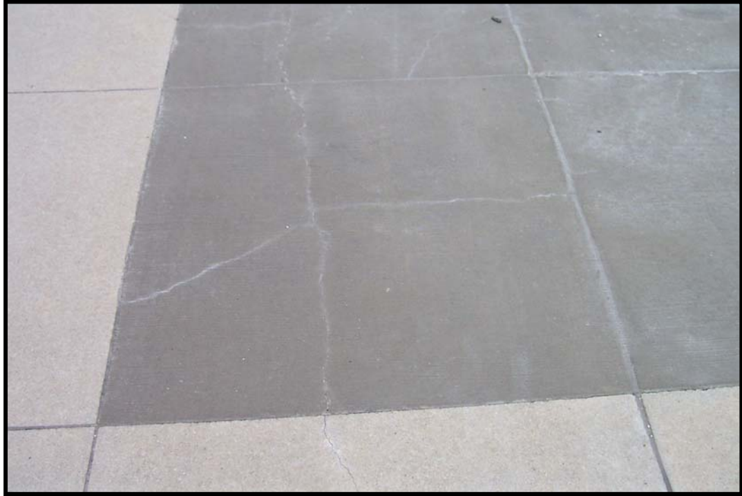
Figure 2.15. All slabs after the second left turn are shattered into three or more pieces.
