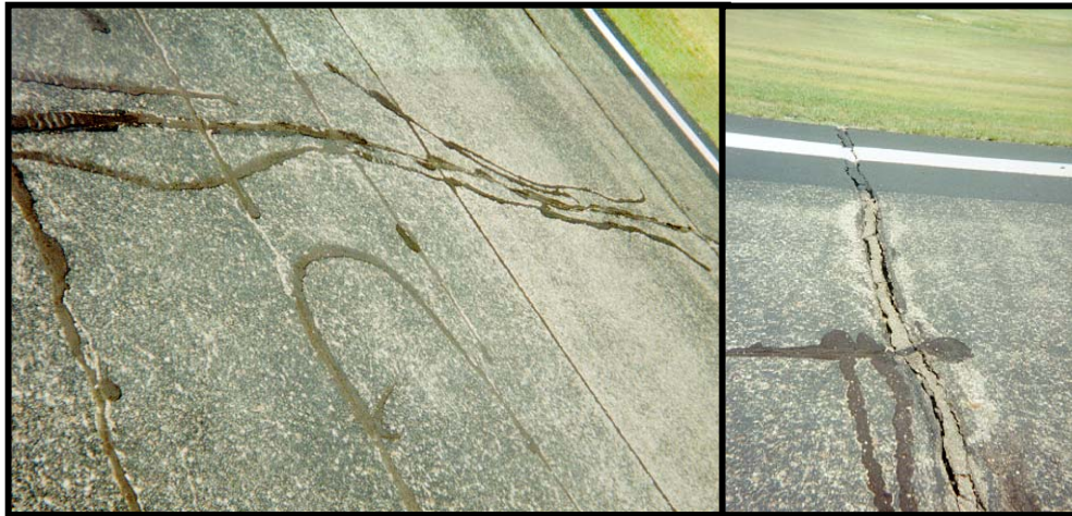
Figure 2.3. Longitudinal and transverse cracking observed at SNH.
