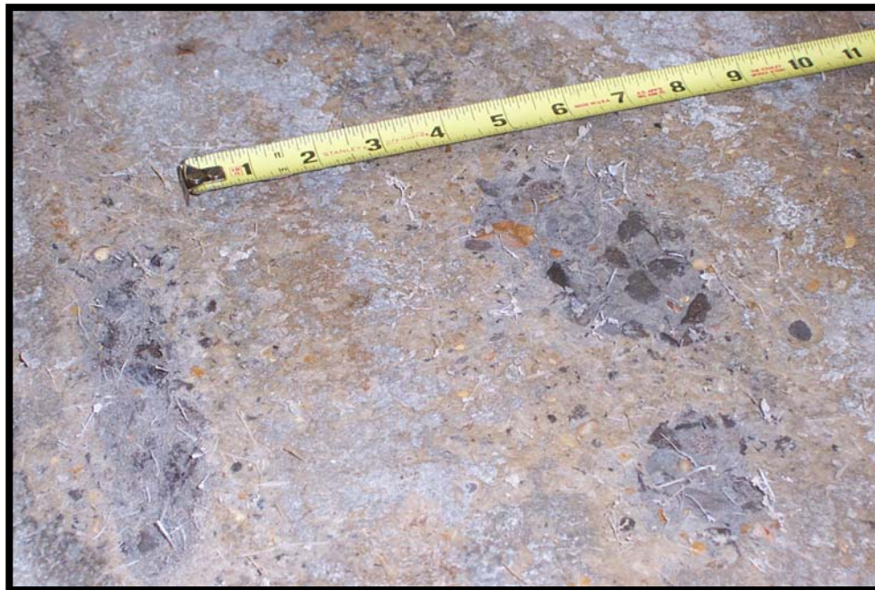
Figure 6.57. Close-up of PCC surface before scrapping with a jackhammer.
