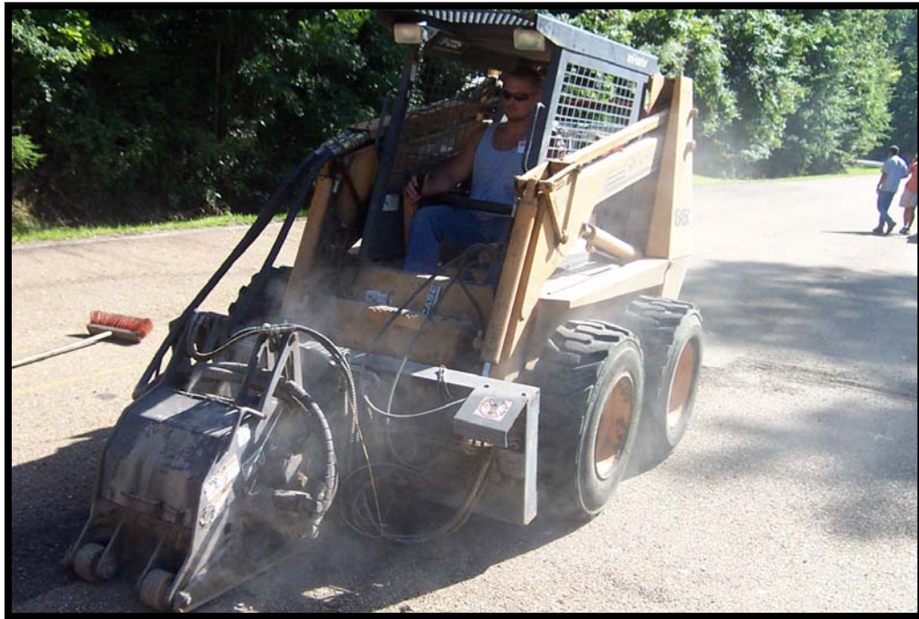
Figure 4.8. A bob-cat ® was used for AC milling at the test section.
