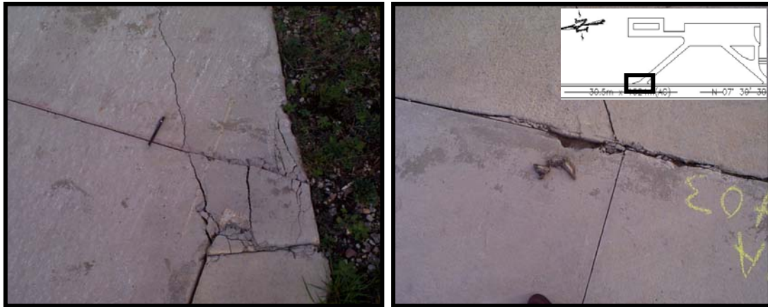
Figure 2.10. Improper joint spacing and slab shapes caused SNH slabs to crack.
