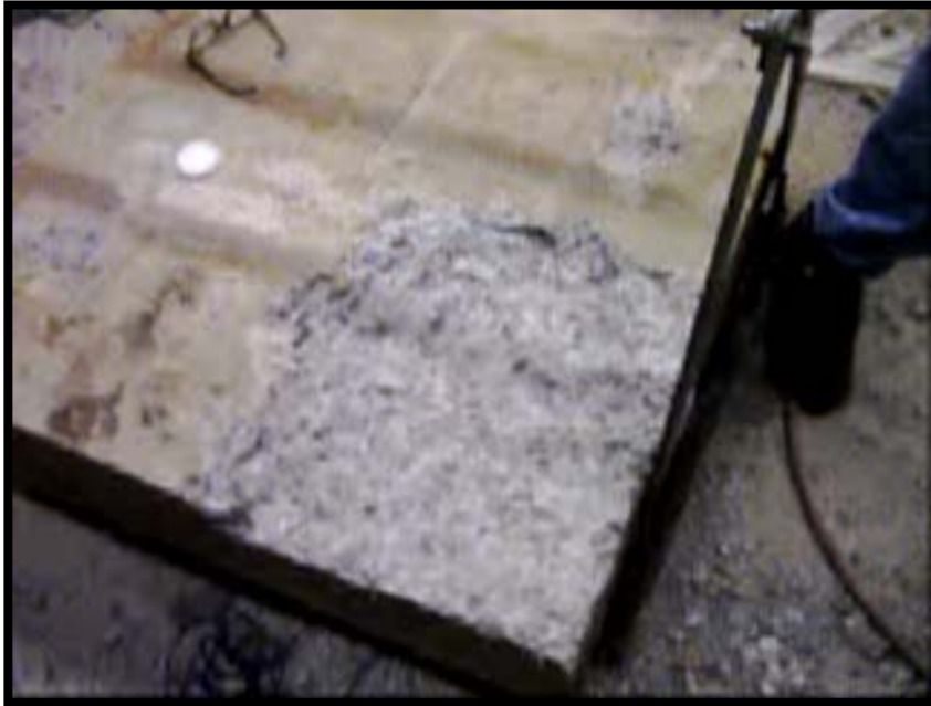
Figure 6.59. PCC surface after cleaning with small jackhammer.
