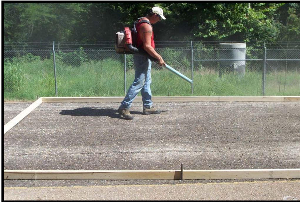
Figure 4.10. Compressed air was used to clean the milled surface at the test road.
