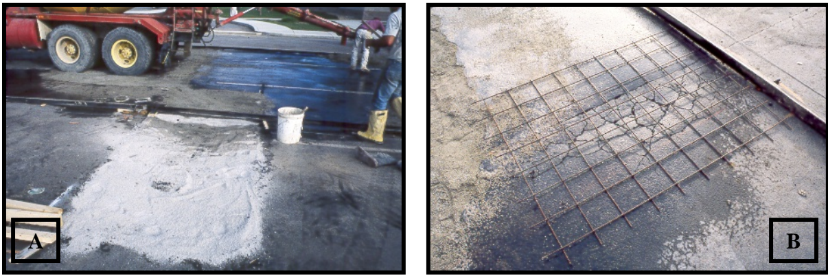
Figure 2.41. Severely distressed areas were repaired before UTW construction.
