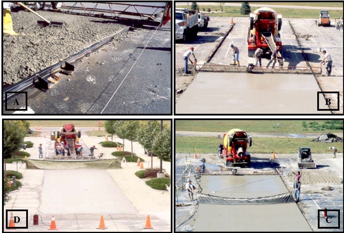
Figure 2.42. PCC was manually placed at church parking lot.
