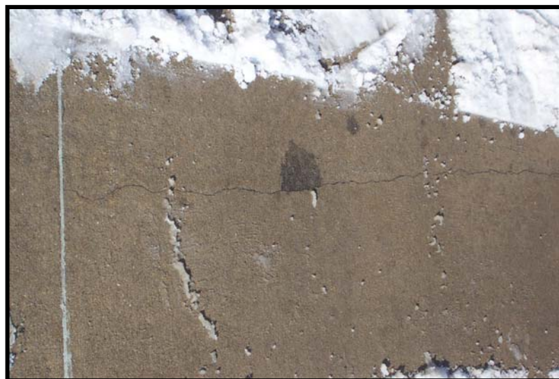
Figure 2.38. A single crack in front of a rear hotel entrance was observed.
