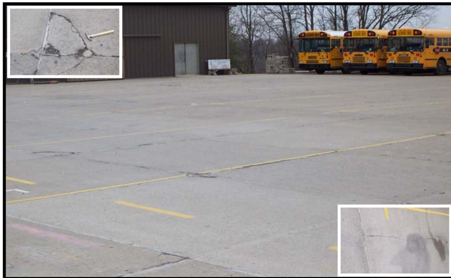
Figure 2.32. Most slabs where buses made turns had broken corners.
