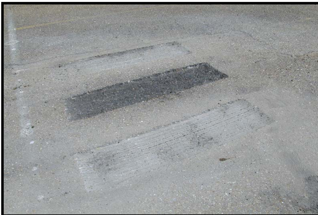
Figure 4.7. After trying three milling depths, a 0.5 inch milling depth was selected.
